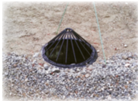
A catch basin fits into a smaller space than a rain garden and traps stormwater otherwise bound for the lake and lets it soak away into the ground. (Courtesy photo)
