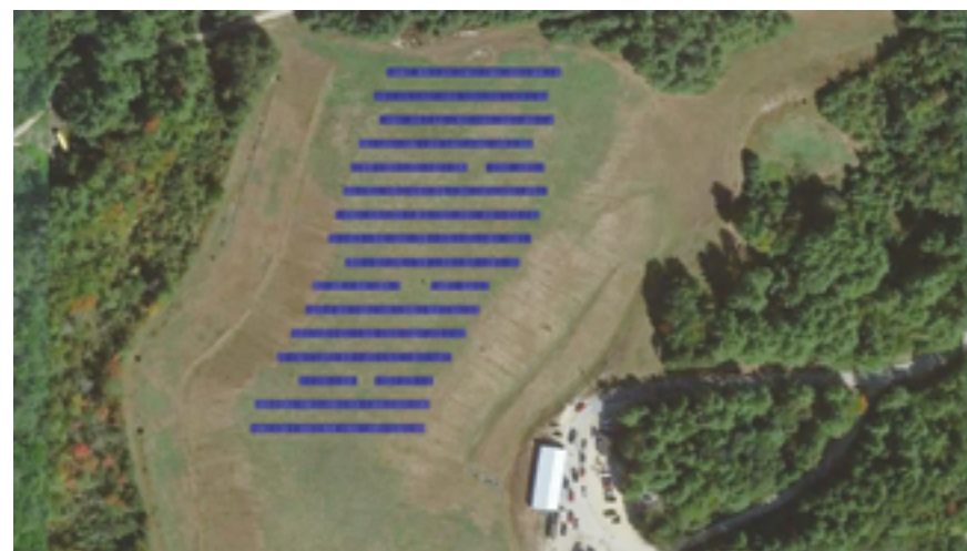
The Jaffrey Community Solar rendition which will be built in New Hampshire in 2024.
