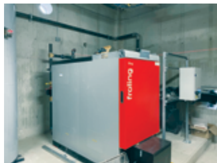
Old Cheshire County Courthouse ( www.courthouses.co/nh/cheshire-cty/ ) opted to have a Froling Energy dried wood chip-fired boiler installed with city gas backup. (Boiler images: Froling Energy)
