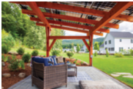
Close up of a SunCommon solar canopy with its bifacial solar panels and handcrafted timber frame. (Photos courtesy of SunCommon)
