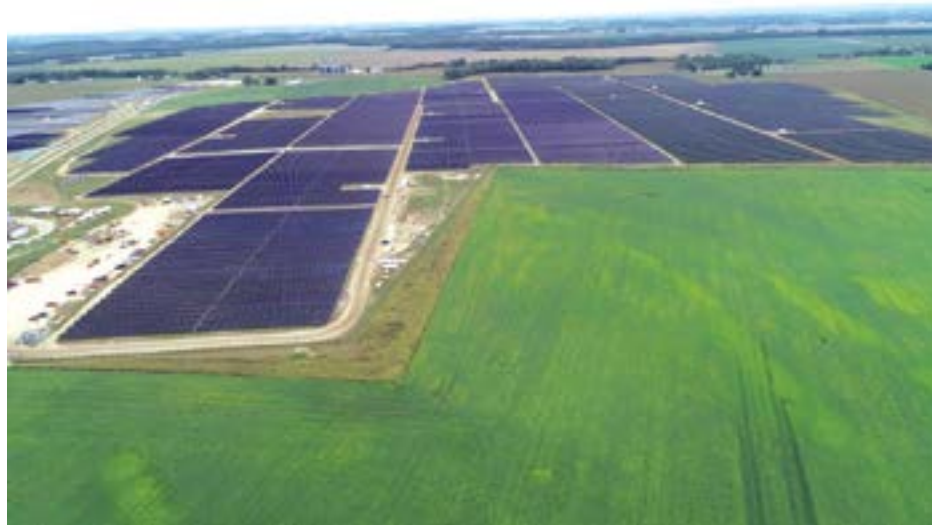
Yellowbud Solar is an operating 274-MW solar photovoltaic (PV) farm in Williamsport, Ross County, Ohio. The farm brings in $90 million in tax revenues for the community and moves Amazon closer to its goal of net-zero carbon emissions by 2040. (Courtesy of National Grid Renewables)
