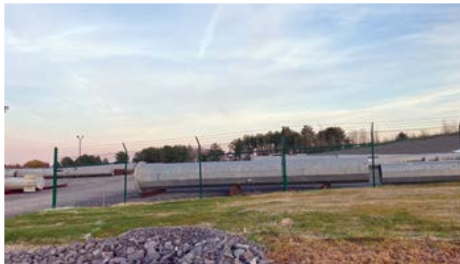
Towers seen from Rt. 20, east of Duanesburg, NY, waiting to be erected as the state continues to improve the grid efficiency in the capital region. (N. R. Mallery)
