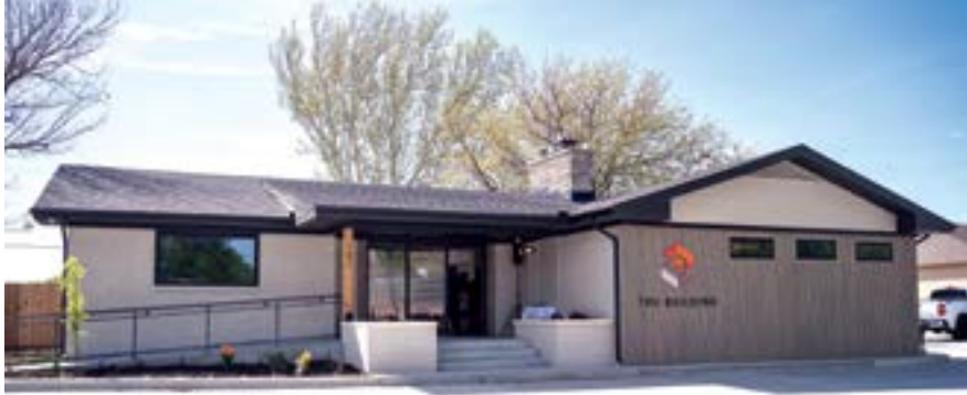
TRU-Building's new headquarters incorporated energy efficiency through the installation of a Taco System M heat pump system seen below. (Courtesy photo)
