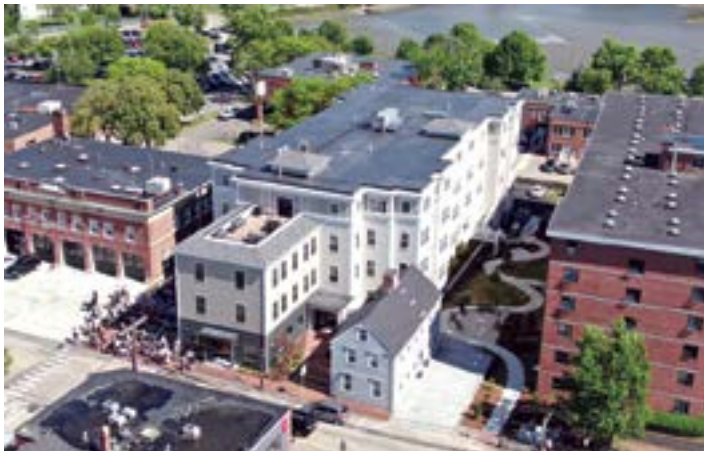
The Ruth Lewin Griffin Place in Portsmouth, NH. The photovoltaic and the ERV systems are located on the roof. (Images from Eckman Construction)
