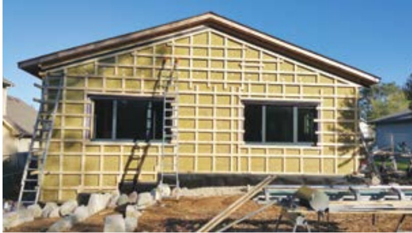
High performance construction with attention to sealing and continuous insulation can help to solve the housing and climate crises at the same time. (kimchi and kraut)
