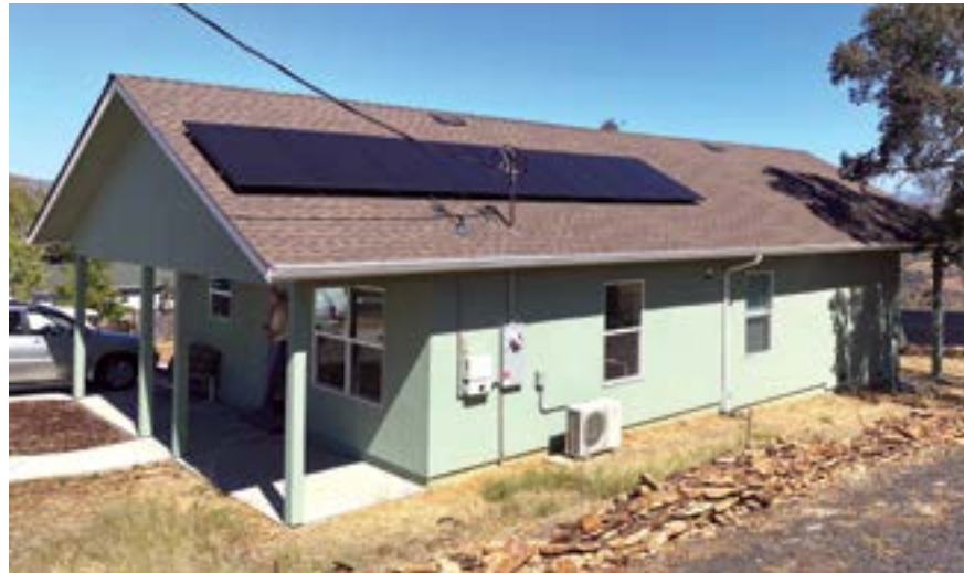
The 1,250 s.f. home features a 2.76kW photovoltaic solar array. The cost to build this pilot project house was $320k, but when built at scale (in a subdivision), the same home will be about $190k major cost savings on framing at scale. (Tom Danielsen)
