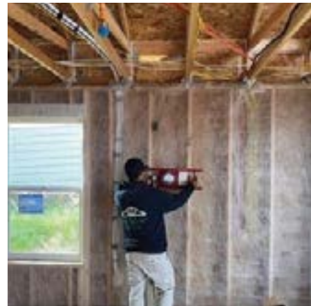
Owens Corning L77 BIB (blown in blanket) insulation was used in the ceilings (R-40) and walls (R-21). (Courtesy image)
