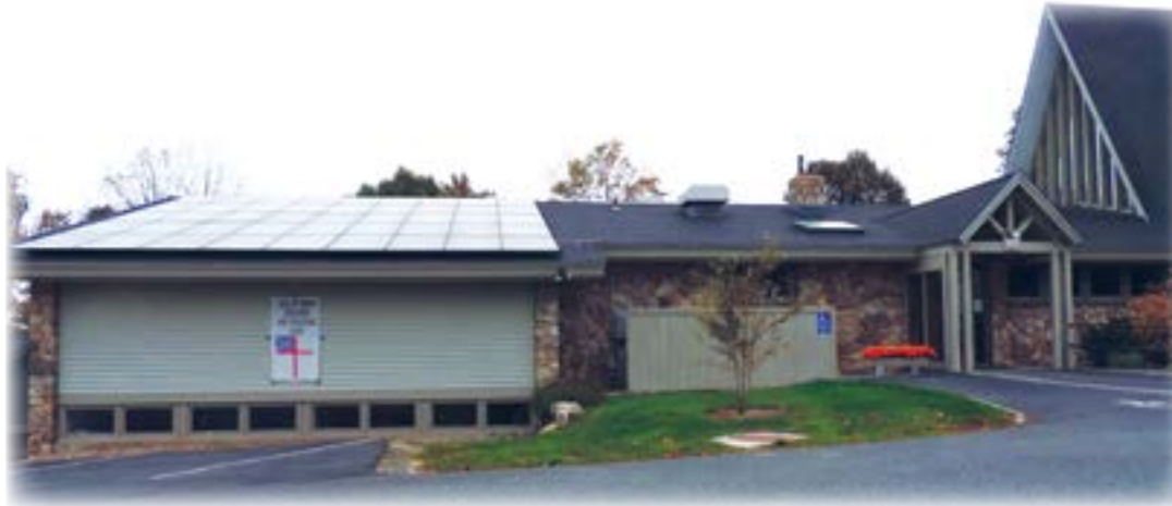
St. Andrew's Church located in New London, New Hampshire reduced their electricity costs by 46% with their 18-kilowatt rooftop solar array. (Larry Chase)
