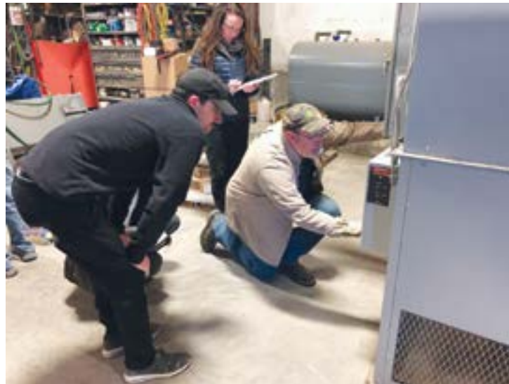
Vermont Tech Renewable Energy student Liam Henchey with Tori Hellwig from the Lamoille County Planning Commission and Nate Brigham from the Village of Johnson collecting nameplate and other information about the buildings' systems during a site visit in March 2023. (Courtesy images)
