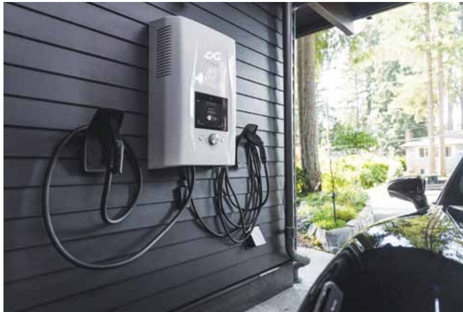
A level 2 charging station set-up in a residential garage operates on 240 volts. This can charge a near depleted battery in three to eight hours depending on the battery size. (pexesl.com)
