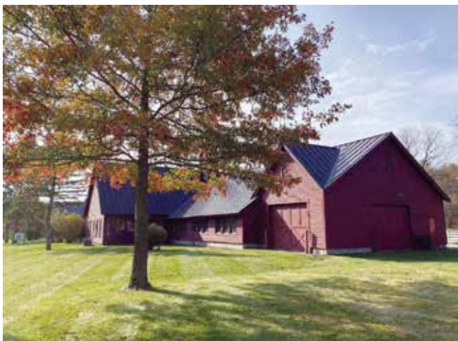
Norwich Farm Foundation's barn. The new roof will hold a 150kW solar array. (Norwich Farm Foundation)
