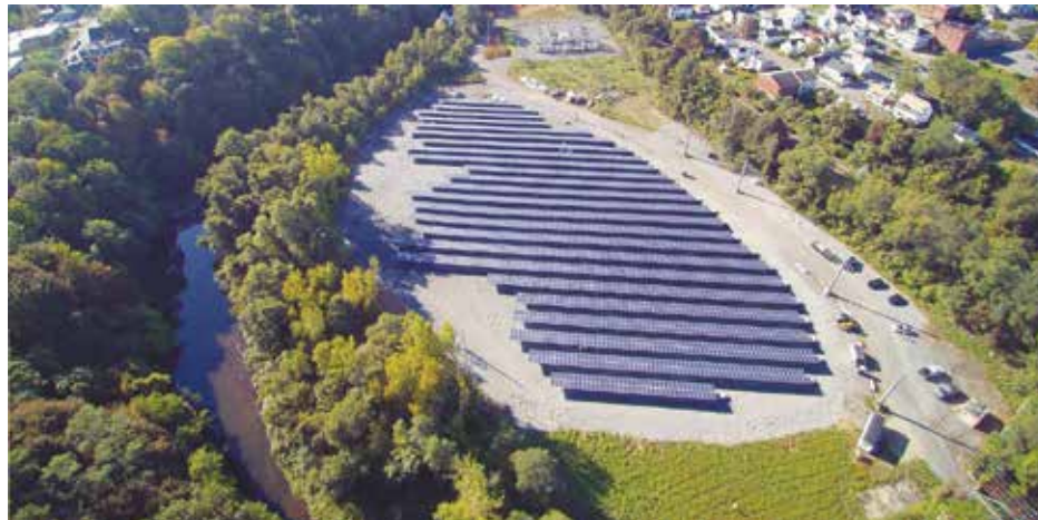
Unitil's Solarway initiative in Fitchburg, MA is a 1.3 megawatt solar array consisting of 3,708 panels. It powers 144 homes. (Unitil)
