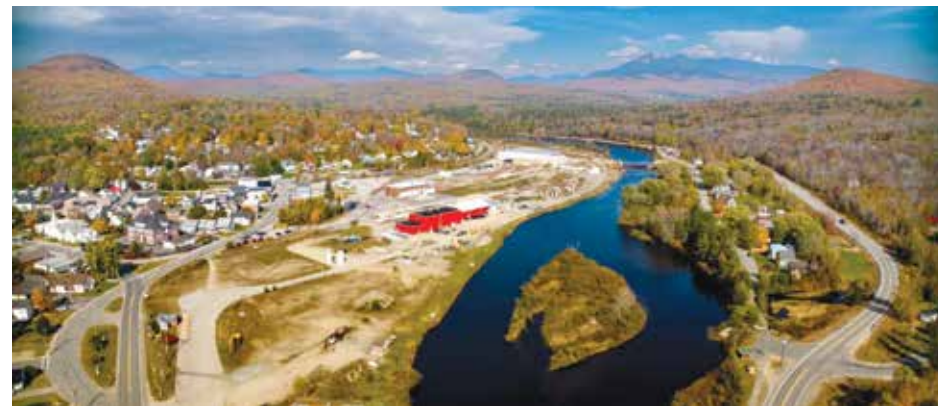
Site of the Q Hydrogen plant in Groveton, New Hampshire. (Q Hydrogen)
