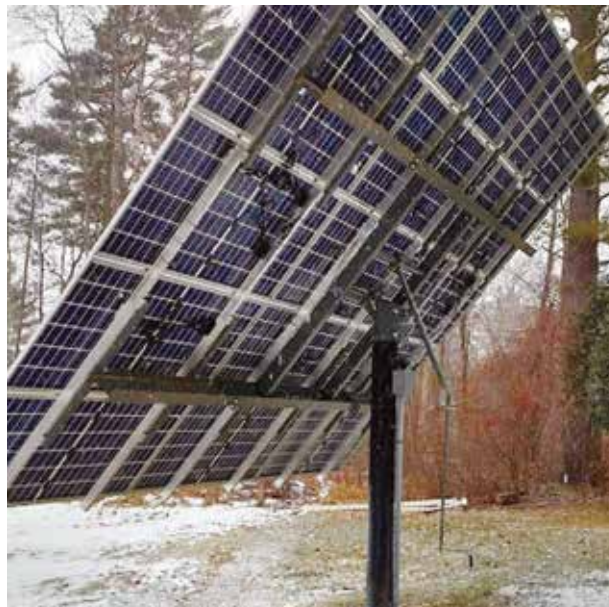
Back of a bi-facial solar array, with an adjustable rack showing a hand crank to adjust the angle. (Courtesy image)
