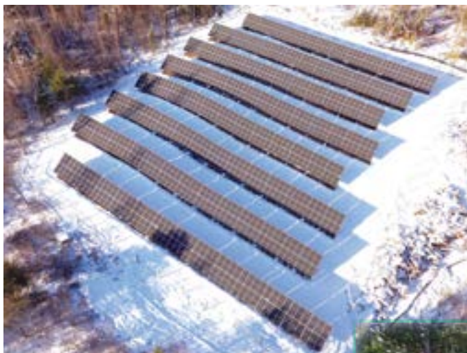
The 344 kW Profile School solar array in Bethlehem, NH. Pictured to the right is Ted Vansant, the owner of New England Commercial Solar Services.
