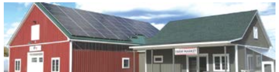
Replenoa Farm's solar array consists of 59 panels producing about 31,600 kilowatt-hours of electricity in its first year of operation. This reduced carbon emissions by 48,938 pounds. (Replenoa Farm)
