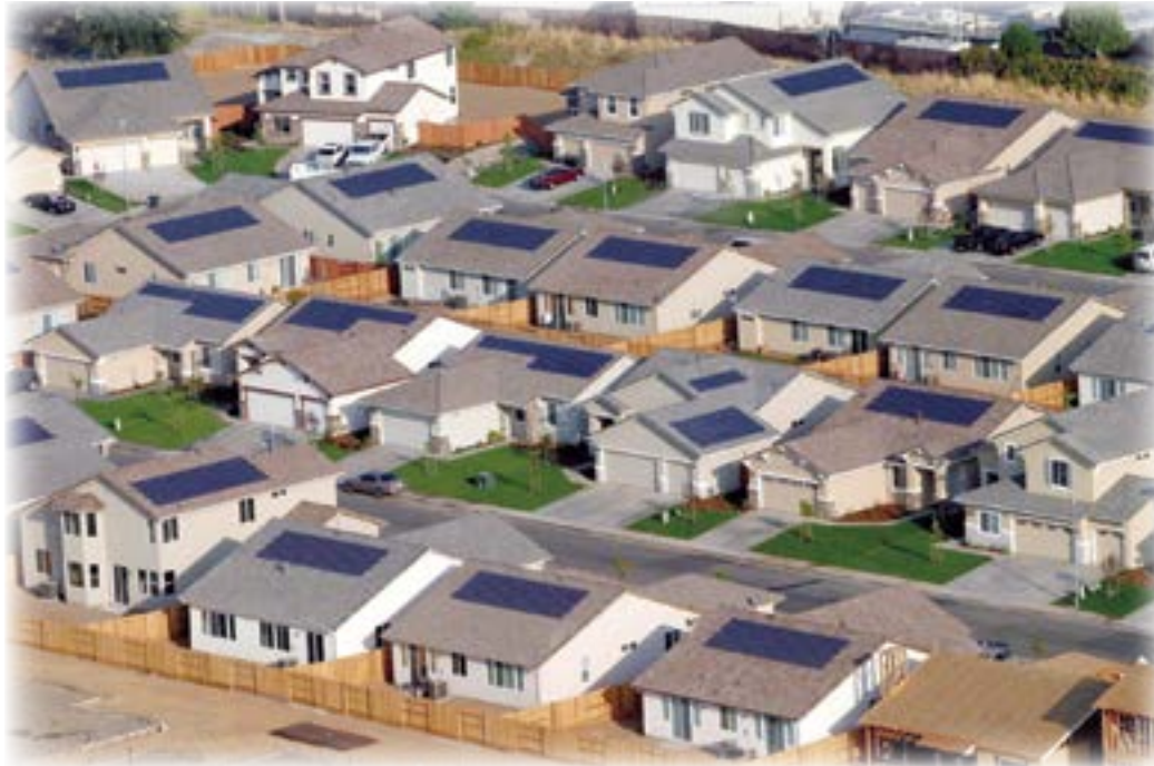
Rooftop photovoltaic panels at Premier Gardens Zero Energy Home Community. As part of the DOE's Zero Energy Homes Initiative, Premier Homes built 95 entry-level houses in Rancho Cordova near Sacramento, California, in 2004. Each is built with advanced energy-saving features and a 2.2 kW photovoltaic system. (Office of Energy Efficiency and Renewable Energy)
