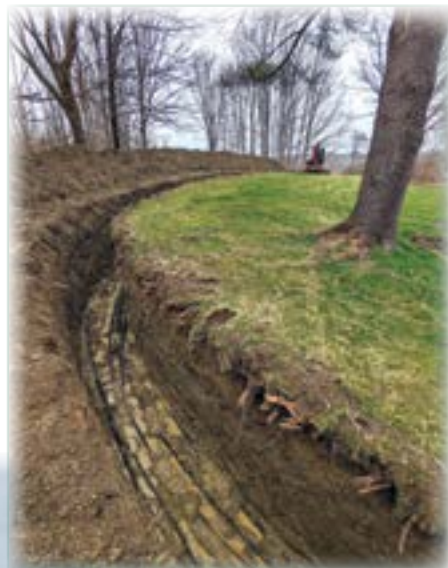
Above: Horizontal geothermal heat exchanger installation in progress. Energy Catalyst offers design and installation of an accompanying geothermal heat exchanger with their heat pumps.
