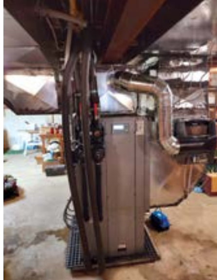
Heat pumps will help NY achieve the goal of prohibiting all fossil fuel heating systems for residential new construction by 2025. This double hybrid heat pump has a heating efficiency over 400%. (Energy Catalyst)
