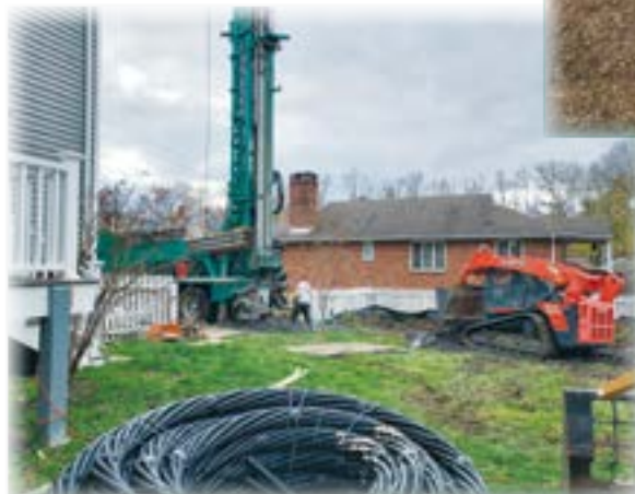
350 ft vertical geothermal heat exchanger being installed by Energy Catalyst. (Images courtesy of Energy Catalyst)
