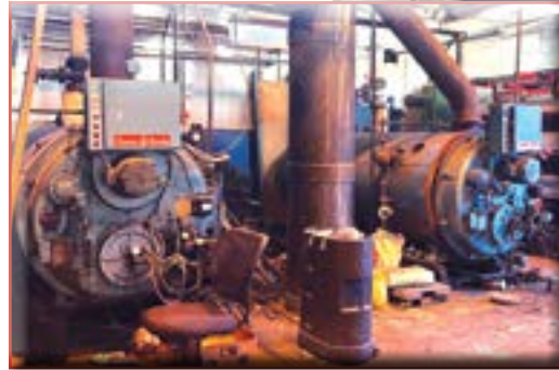
Above: A new high efficiency dried wood chip boiler was installed at 310 Marlboro Street in Keene, NH resulting in a 15% reduction in fuel use while the building occupancy rate went up 60%. The new boiler is a Schmid UTSK with 500 kW or 1.5 million BTUs/hour peak output. Left is the 1961 vintage steam boiler that was replaced. It had a maximum output of 2.4 million BTU per hour and consumed 19,415 gallons of oil per year. (Froling Energy)
