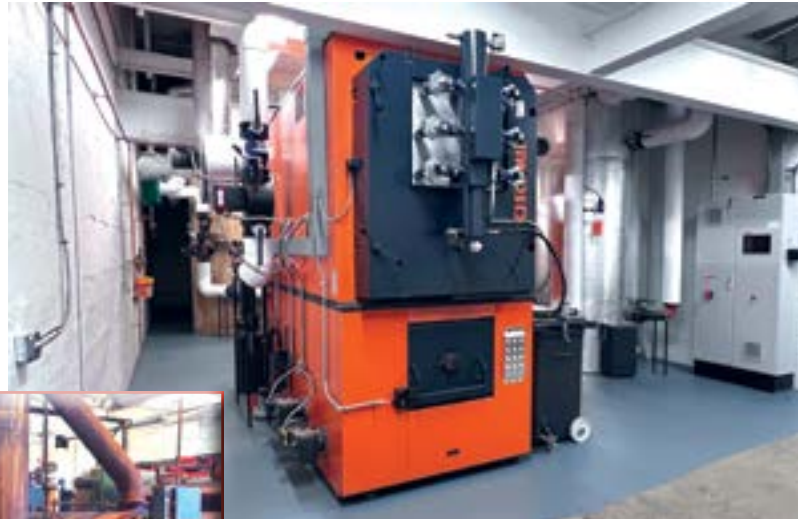
Above: A new high efficiency dried wood chip boiler was installed at 310 Marlboro Street in Keene, NH resulting in a 15% reduction in fuel use while the building occupancy rate went up 60%. The new boiler is a Schmid UTSK with 500 kW or 1.5 million BTUs/hour peak output. Left is the 1961 vintage steam boiler that was replaced. It had a maximum output of 2.4 million BTU per hour and consumed 19,415 gallons of oil per year. (Froling Energy)
