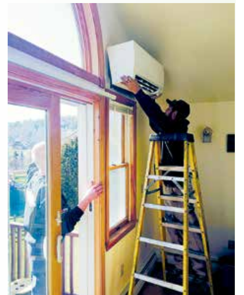
Installing an air-source heat pump will help this homeowner use half the energy needed for propane and oil systems. Photo: Steve Costello, GMP.
