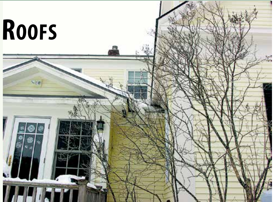
Converging roofs led to snow and ice accumulation which caused interior wall leaks.
