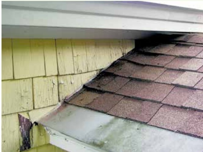
A "kick-out" at the bottom of the roof would prevent the saturation of the siding.
