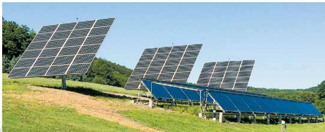
Left: Rob Head's family home in Burlington Flats, NY is powered by 100% renewable energy. Above: The PV solar tracking system sits above the solar thermal evacuated tube arrays. Courtesy photos.
