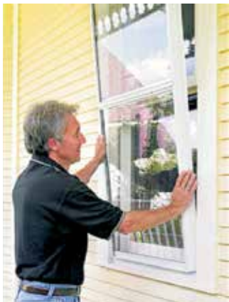
Storm windows, such as the interior unit shown here, can be custom ordered from window distributors and some big box retailers. Some common sizes are available off the shelf.
