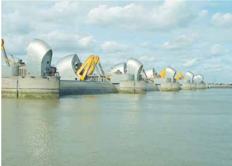
The Thames Barrier protects London against flooding. At the time of its construction, the barrier was expected to be used two to three times per year. It is now being used six–seven times per year. Photo by Andy Roberts. CC BY-SA 2.0
