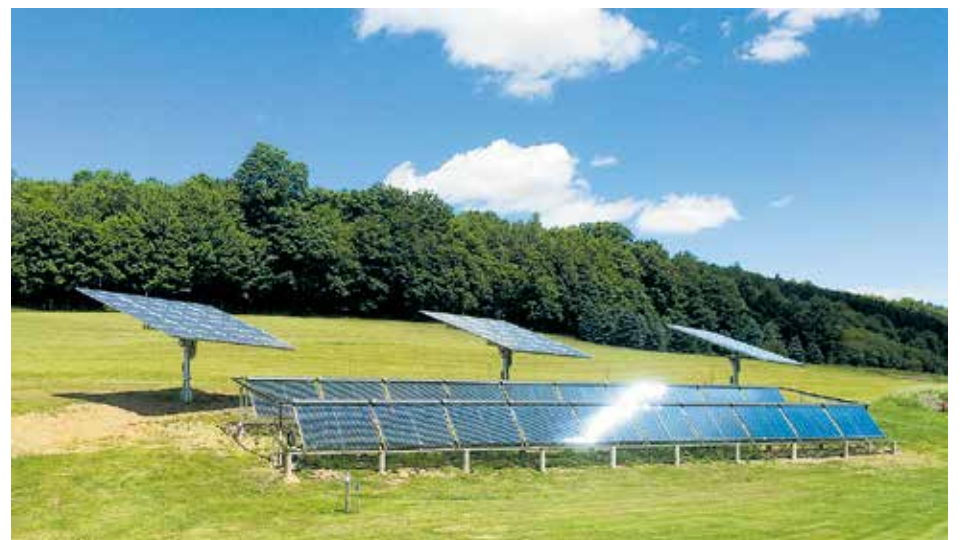
Left: Rob Head's family home in Burlington Flats, NY is powered by 100% renewable energy. Above: The PV solar tracking system sits above the solar thermal evacuated tube arrays. Courtesy photos.
