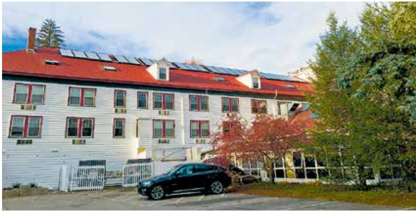
Eastern Slope Inn solar thermal. Photo courtesy of Revision Energy.
