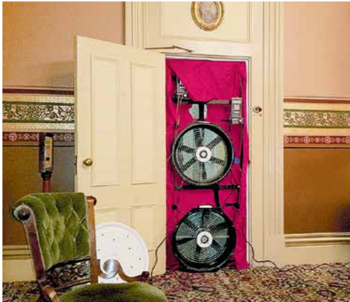
Double blower door test at the Statehouse by Common Sense Energy. Photo: Allan Bullis.
