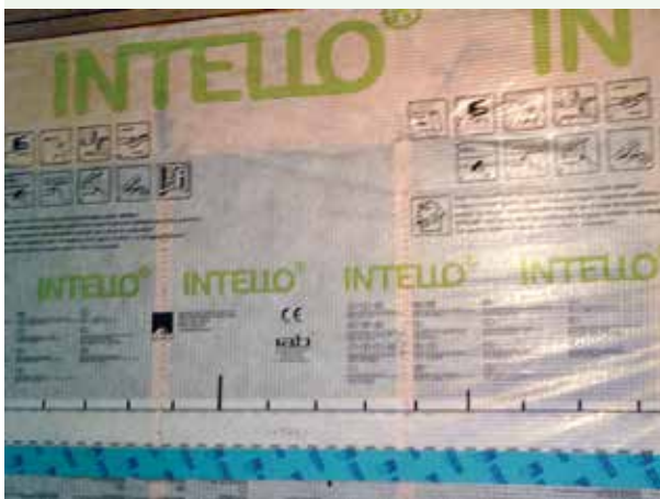
Interior smart vapor retarding membrane. Photo by Michael Goetinck
