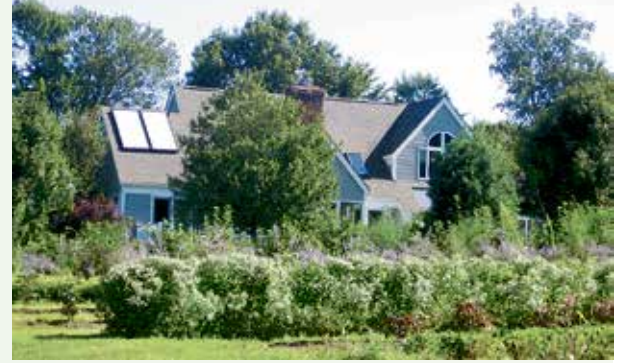
Chardes House High Meadow Farm with a solar thermal (hot water) system on the roof, in Warwick, New York. Photo courtesy of NYSES.
