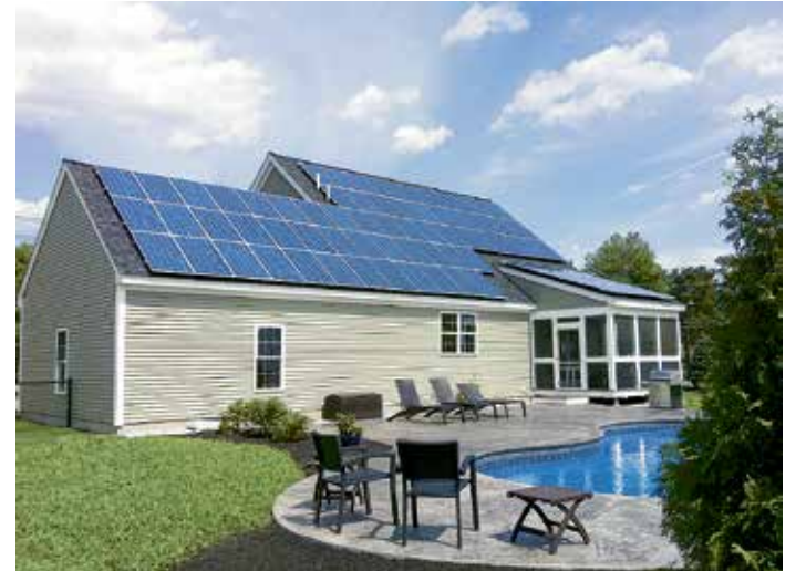
Transformation's award winning custom house at 14 Cavite St., Devons Green, MA. Photo courtesy of Transformations Inc., Townsend, MA.
